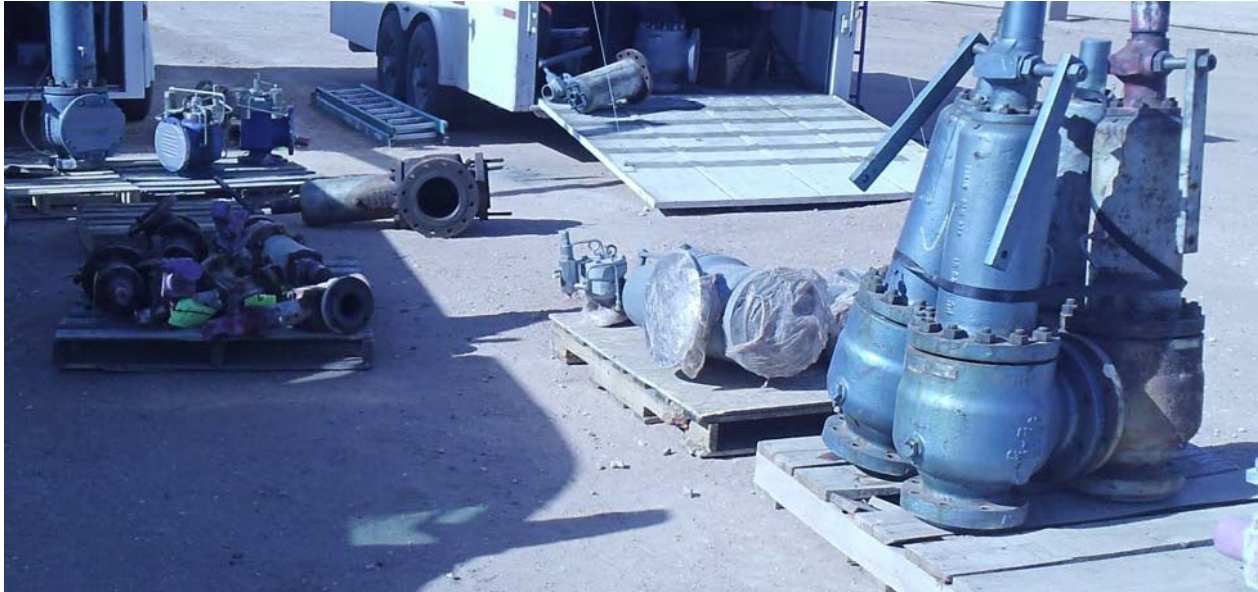
Figure 37—Example of Improper Storage of Valves
